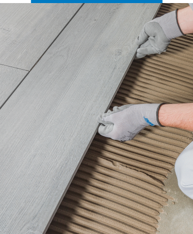
Installation of wood-effect tiles on a substrate waterproofed with Mapelastic
